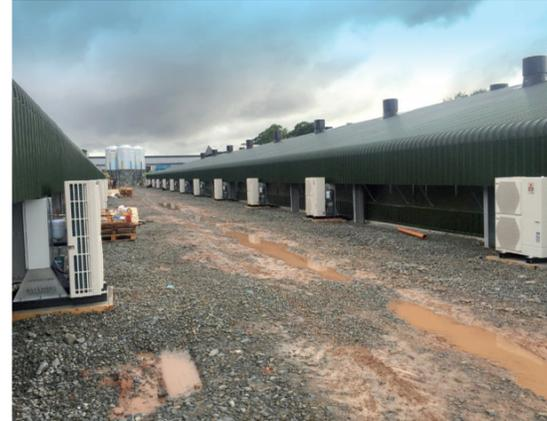
ABOVE: 24 Air source heat pumps on the new sheds have proved much cheaper to run than the existing Biomass.
